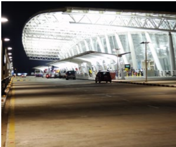
Chennai International Airport, India
