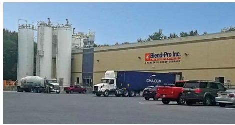
Penetron/Blend-Pro Manufacturing Facility, Allentown, Pennsylvania, USA
