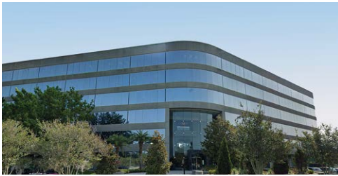
Penetron International Headquarters, Orlando, Florida, USA
