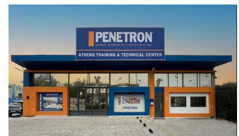
PENETRON HELLAS Facility, Athens, Greece
