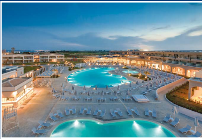
SWIMMING POOL SYSTEMS
