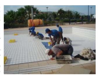
B. In case there are failures in the topping surface of the existing pool, with tiles or chippings and there are cracks and water loss, the tiles or chippings should be removed, the cracks should be repaired with repairing mortar and the concrete should be repaired with crystalline waterproofing coating.
