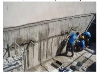
areas. When PENECRETE MORTAR® has been set, but is still moist, apply a second layer of PENETRON® slurry coat, on the repaired areas.
