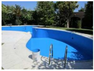
Furthermore, the SEALCOAT<sup>TM</sup> SYSTEMS can be reinforced with a fiberglass grid between layers (mesh 5x5 mm). In that type of application, place the grid on the first layer, while wet, and fully cover the grid with the second layer, on the next day. The use of fiberglass grid is expected, to increase the total coverage of the system, up to approx. 0.6 lb/ft² (3 kg/m²) in 2 layers.
